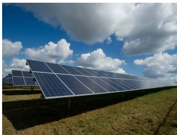
Solar development on Langland Farms in Coopersville.
